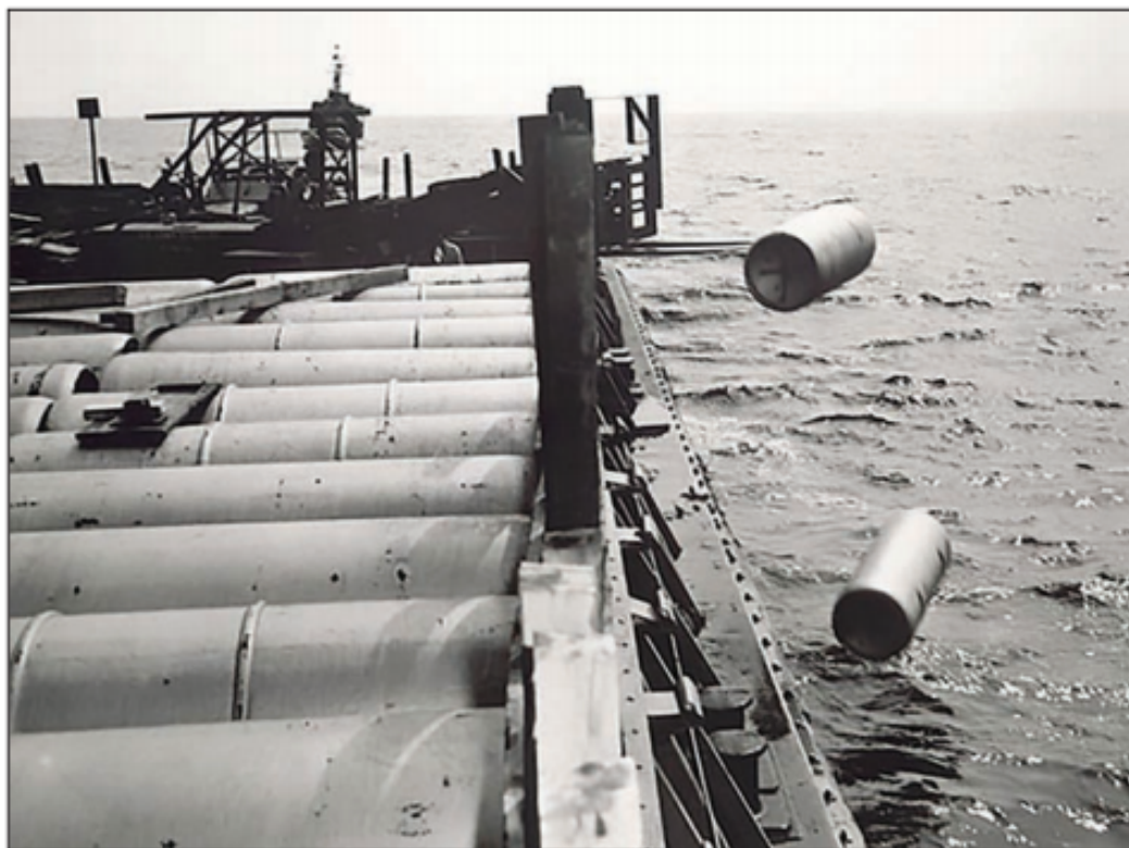
Photo 1. Conducting sea disposal operations. Photo courtesy of the U.S. Army.
